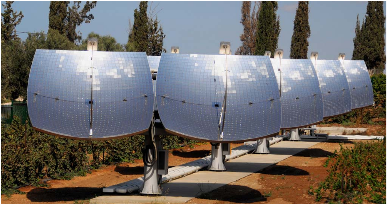
ZenithSolar Z20 CHP Solar Technology
